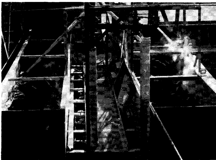
Gel conditioning troughs of 600-ton-per-day pear waste plant, operating on the 1952 crop. The installation was built and is operated by Pacific Biochemical Co. from design developed by Western Regional Research Laboratory
